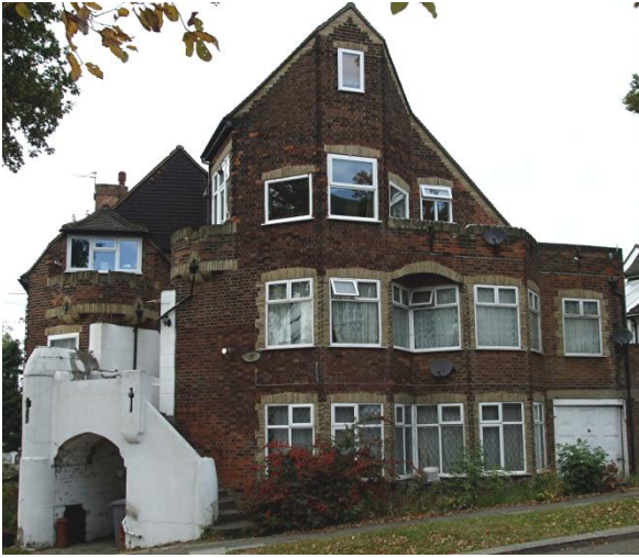
Stonegate Court in Buck Lane. [Photograph by Philip Grant, 2009]
